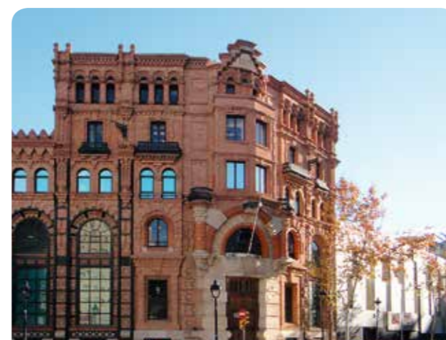
Renovation associating the ancient and the modern: older part renovated
