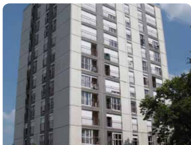
Before the renovation
