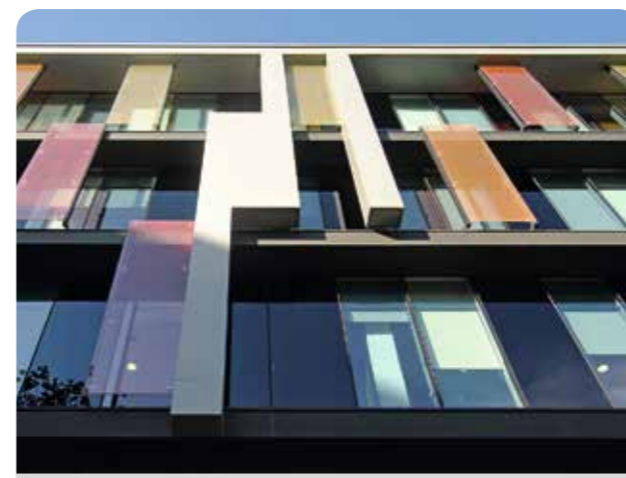
After the renovation
